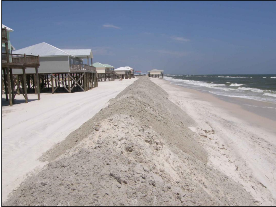
Figure 5. Second emergency sand pile constructed along the beach in response to the BP/Deepwater Horizon oil spill to keep oil on the beachface (photo date: May 12, 2010). This feature was mechanically removed by February 2011.
