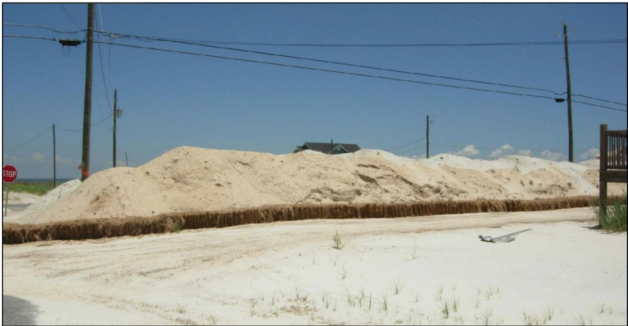
Figure 4. First emergency sand pile constructed south of Bienville Blvd. in response to the BP/Deepwater Horizon oil spill to keep oily water from overwhelming the entire island into Mississippi Sound (photo date: June 24, 2010).
